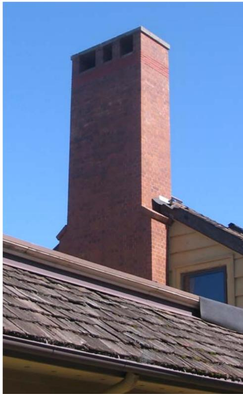
*New chimney built before the old roof was removed*
